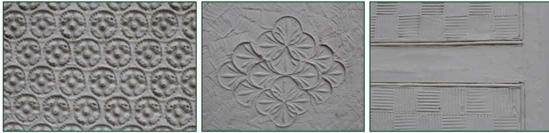
Figure 14 Examples of rendering and simple pargetting in Much Hadham
